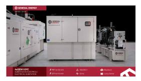
A special canopy with sound attenuators and a 1.300 L fuel tank for 72 hours of autonomy – at 75% load – is one of the features of the genset we've designed for different substations in Zaragoza.
